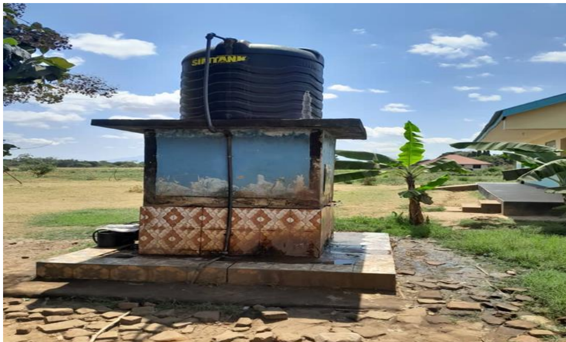
Photograph 3: Water tank connected to a borehole and a tap at School B primary school
