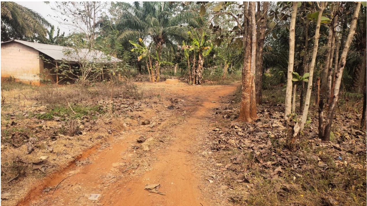
Plate 2: Showing access road in Esa Oke farm settlements.
