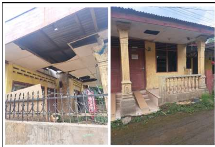
Figure 4: Existing Roof Condition
