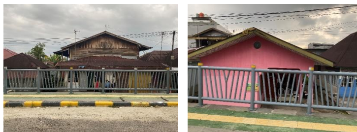
Figure 14: Road conditions are higher than the buildings on Perdagangan Street
