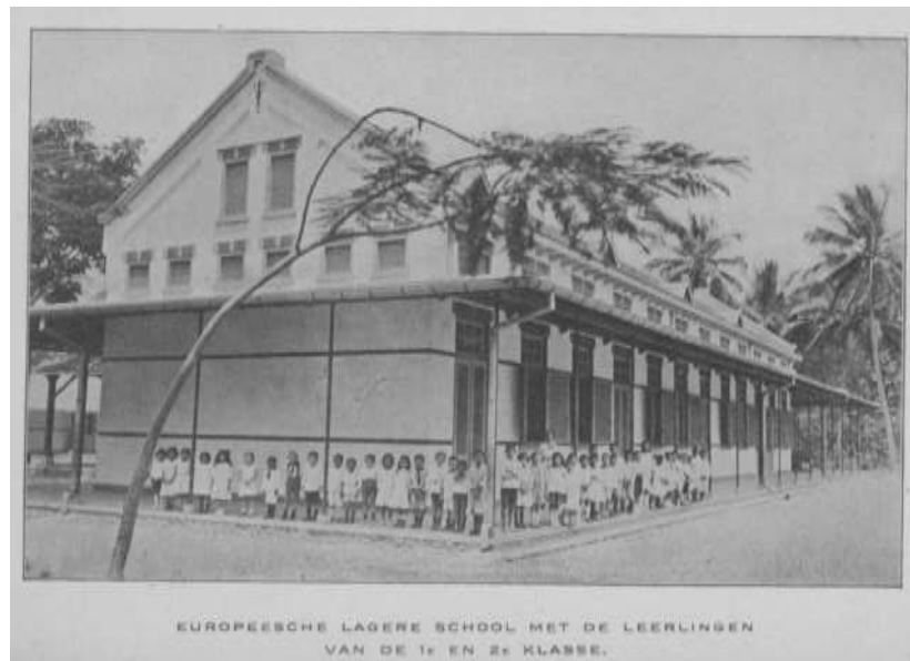
Figure 3: The Condition of SCS's ELS in Tegal [24].
