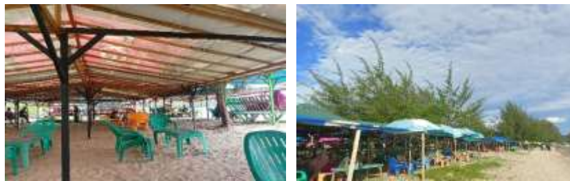
Figure 1: Huts/resting places built without proper planning and design
