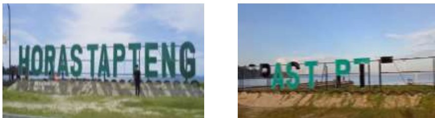
Figure 5: Damaged "Sign Horas Tapteng" sign
