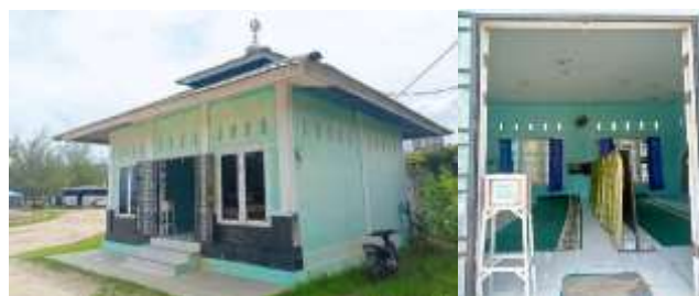
Figure 9: Condition of the mosque
