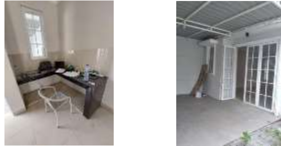
Figure 4.10 windows and back doors for air circulation out of the kitchen Source: Personal Sports, 2023
