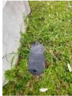
Figure 4.11 Citraland Gama City Building Water Meter Source: Private Sports, 2023
