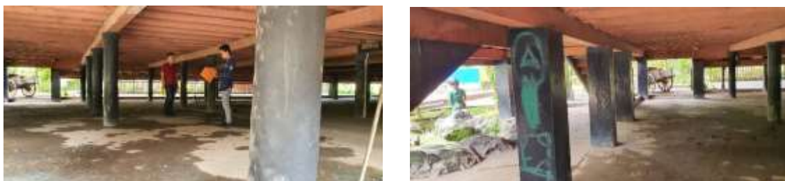
Figure 4.5: Bantayo Poboide Traditional Building Support Poles
