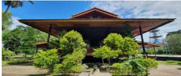
Figure 4.1: Front View of Bantayo Poboide Traditional Building
