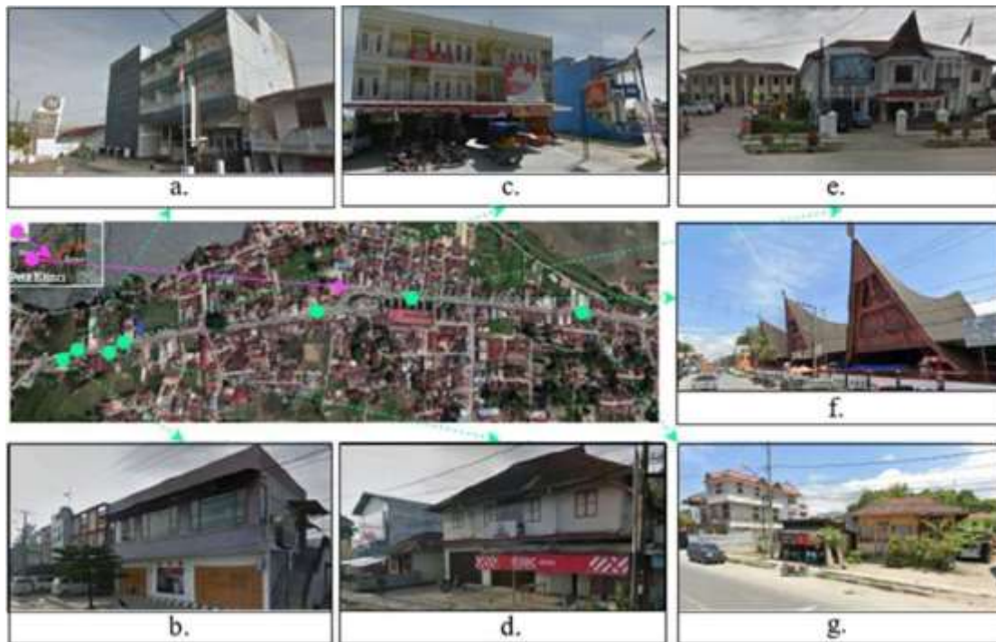
Figure 4.4 Physical Condition of Arterial Road Corridor Building in Balige District
