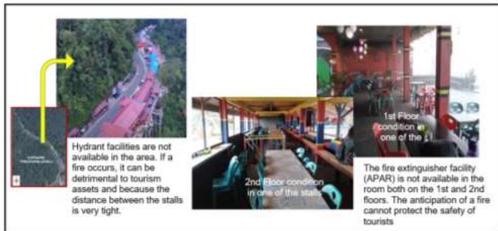
Figure 4: Inner condition of shop
